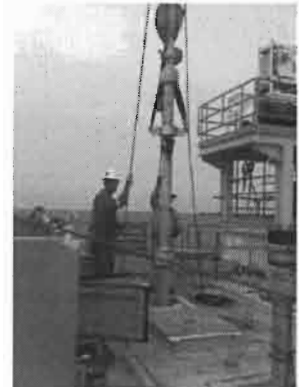
Lowering/raising slickline and wireline perforation tools
